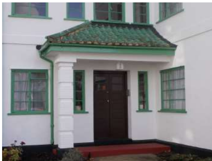
Figure 50: One of the three front entrances to Pinner Court
