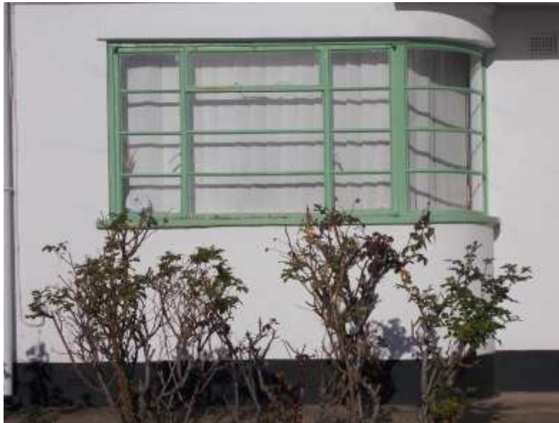
Figure 78: Typical Crittall window to both Pinner Court and Capel Gardens
