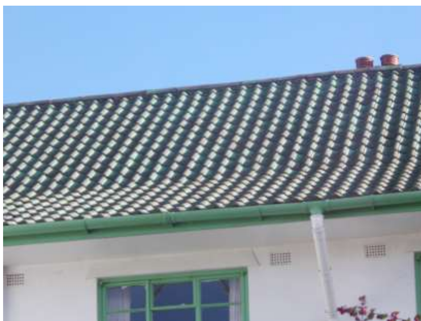
Figure 49: Typical pan tiled hipped roofs with sprocketed eaves of Capel Gardens
