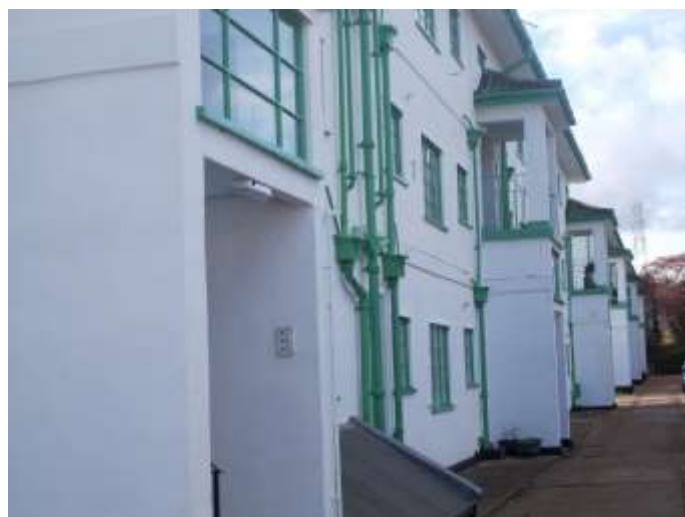
Figure 51: Rear servants' entrances in projecting two-storey loggias to Pinner Court
