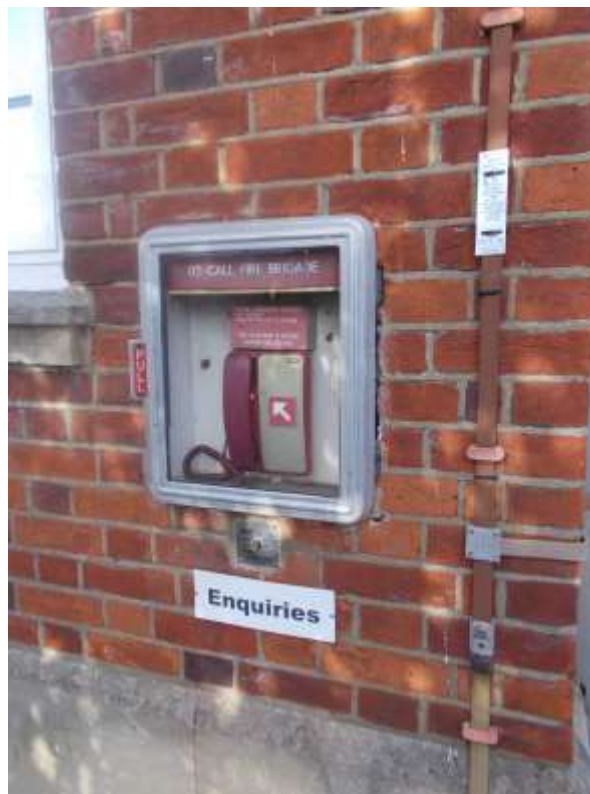
Figure 62: Good original fire station call box feature to frontage
