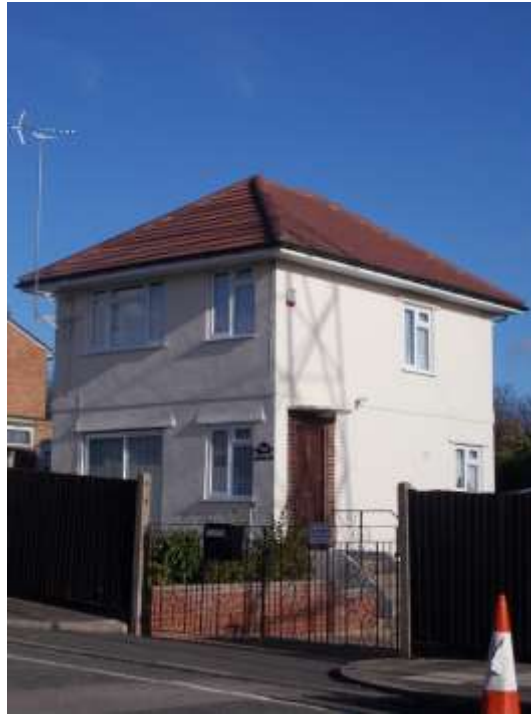
Figure 110: Modernist inspired features of the Lodge include its smooth render finish, and raised geometrical render banding
