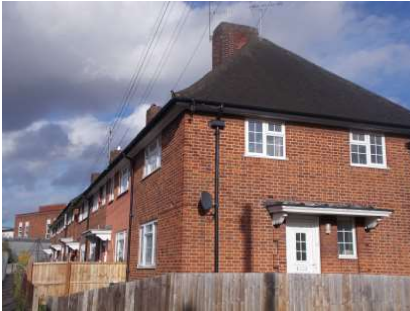
Figure 68: Workers' cottages to firestation – open decorative porches provide continuity and regularity to the design
