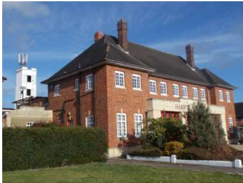
Figure 26: Landmark quality of the Harrow Fire Station and training tower behind with plentiful greenery in front
