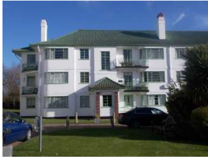
Figure 10: One of the western blocks to Capel Gardens, Pinner Road built 1935-37
