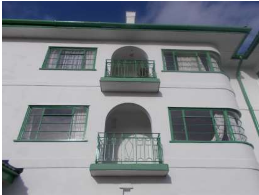
Figures 46 and 47: Typical geometrically designed balconies to Pinner Court some of which include recessed elements
