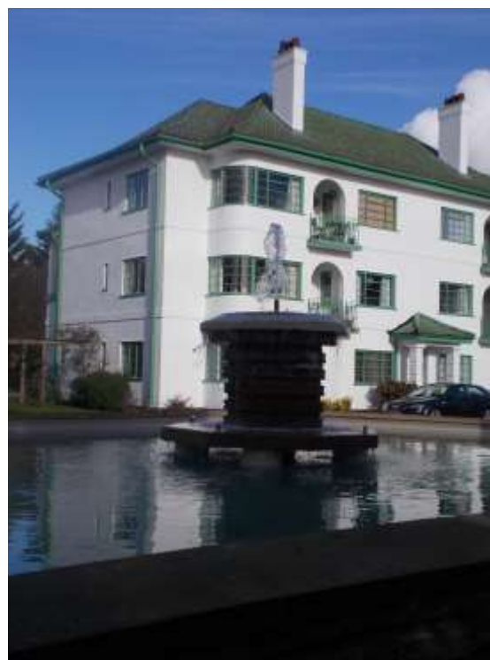
Figure 59: The geometrically designed ornamental garden to Pinner Court, with listed fountain centrepiece, complements the Art Deco building
