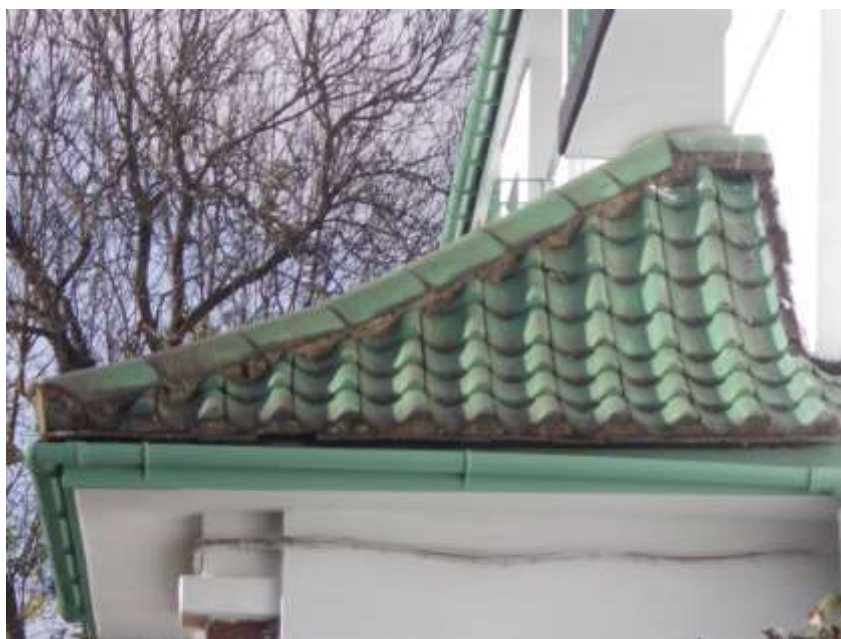
Figure 48: Typical pan tiled hipped roofs of Capel Gardens are part of the colonial/hacienda style
